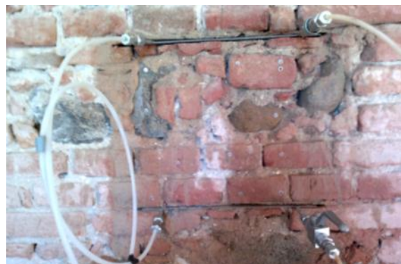
Double flat jacks test
