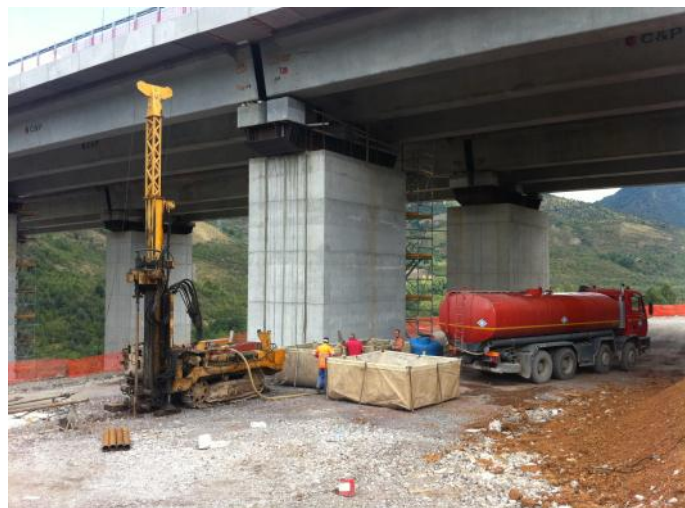
Drilling operation for inclinometer and piezometer installation
