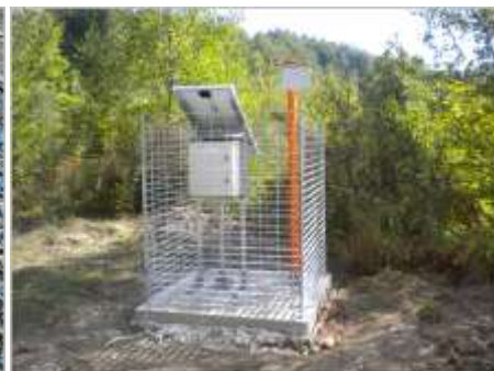
GPS measurement station
